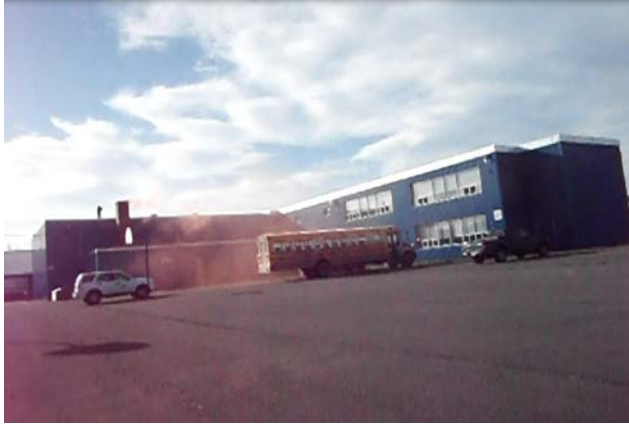
Photo 1: Showing smoke emitter deployed in Test No. 3 at 13:34 minute mark. Direct reading instrument at Location 3 on lower mechanical room roof measured CO concentration of 0.2 ppm during the same time this still frame was captured.
