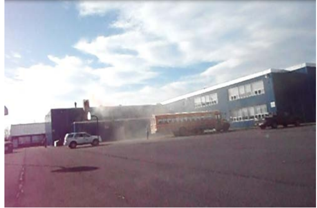
Photo 2: Showing smoke emitter deployed in Test No. 3 at 13:35 minute mark. Direct reading instrument at Location 3 on lower mechanical room roof measured CO concentration of 0.1 ppm during the same time this still frame was captured.
